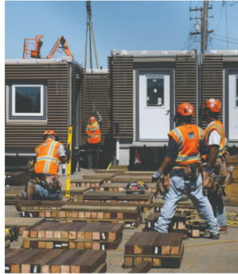
The Watsonville tiny home village is now under construction behind Westview Presbyterian Church, located near the Pajaro River. The 32 modular units can temporarily house up to 34 people.
